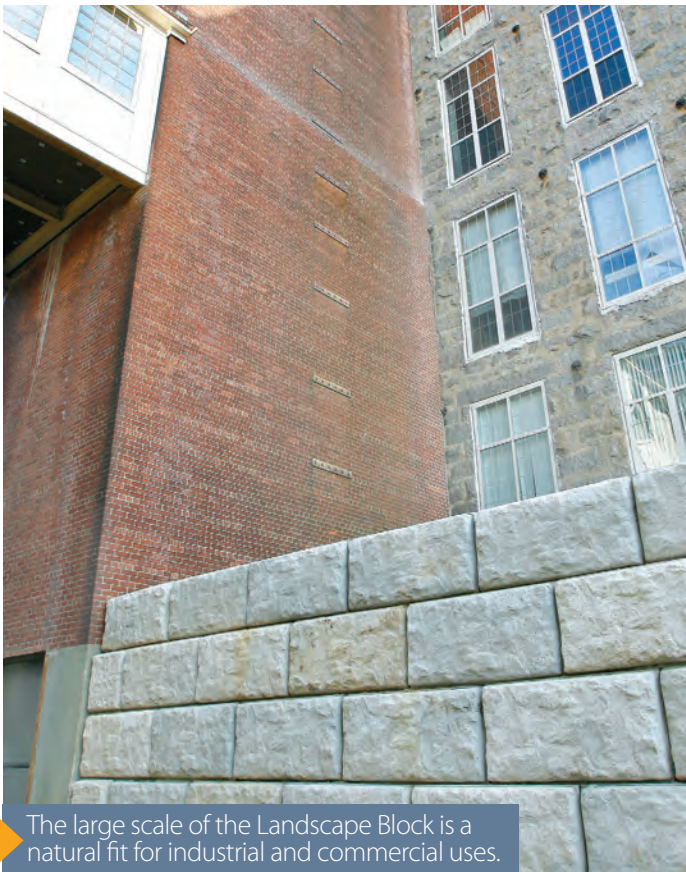
Landscape Blocks have been engineered to hold back a lot of earth.
