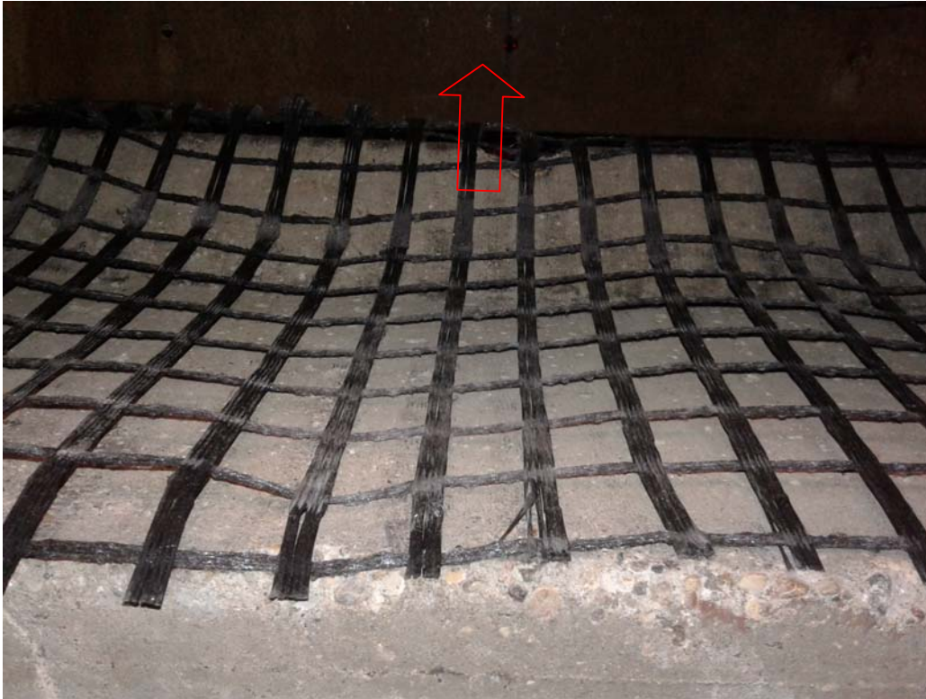
Figure A-5. Abrasion and rupture of geogrid at the completion of a test. The arrow points to direction of connection load.
