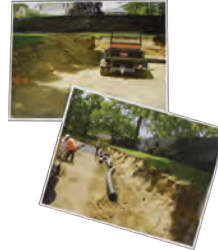
Photos of future retaining wall site
