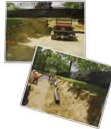
Photos of future retaining wall site
